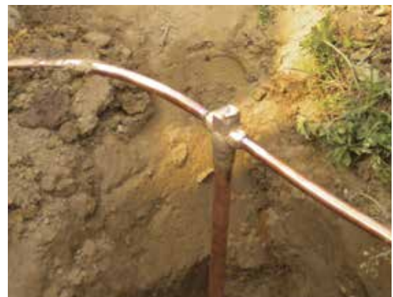
GT Cadweld connection
